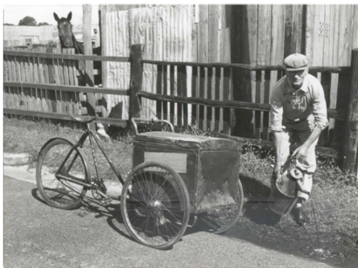
Oil equipment used against mosquito larvae. Brisbane City Council, date unknown.
